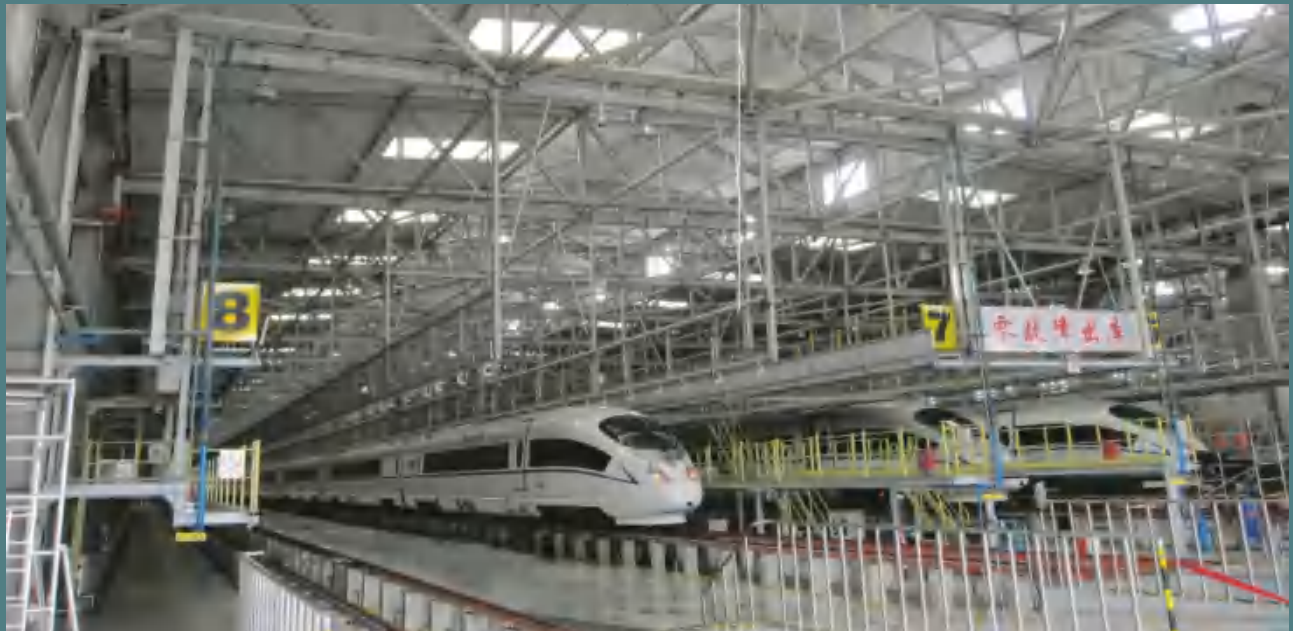
Bullet Train Maintenance Shop
